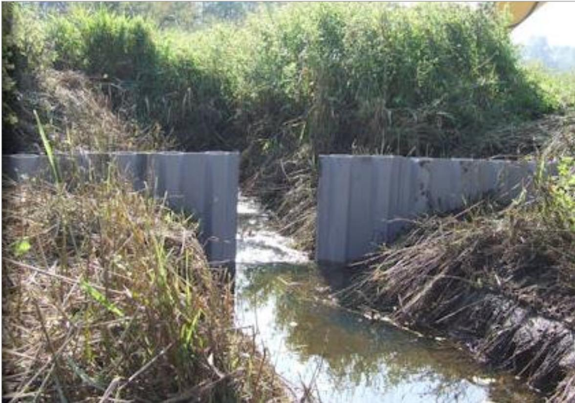
Figure 5.7 Partially blocked drain, with level of blocking determined by driving plastic piles in the centre of the drain further into the peat © David Coley (The Plastic Piling Company)
