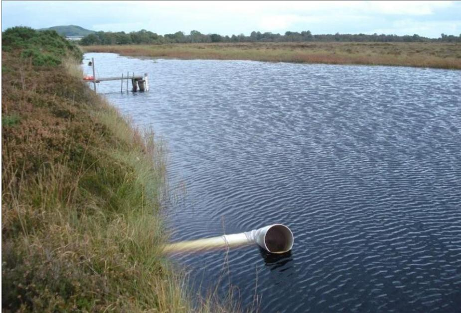
Figure 5.14 Photo of the successful large high bog bund at Raheenmore Bog SAC illustrating need for ongoing maintenance and water level control © NPWS
