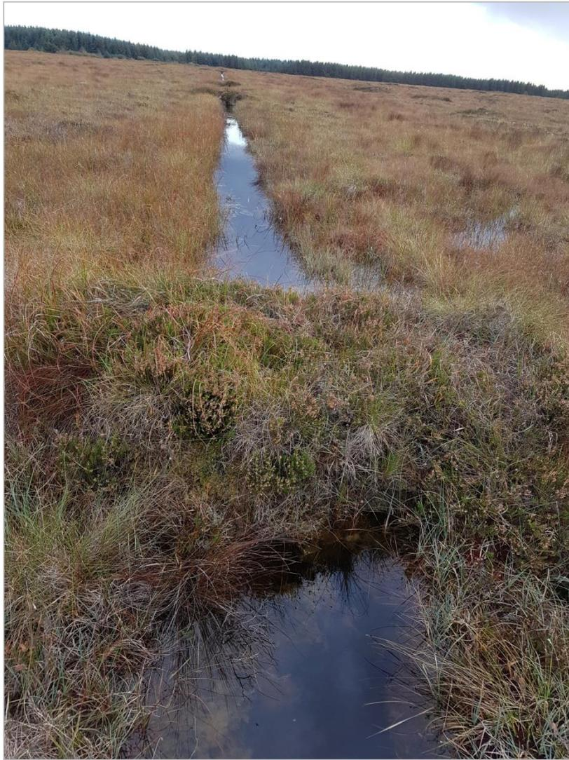
Figure 5.2 Example of a peat dam at Moyarwood Bog, Co. Galway. Note the water table has risen to the surface within the drain and adjacent areas © Francis Mackin
