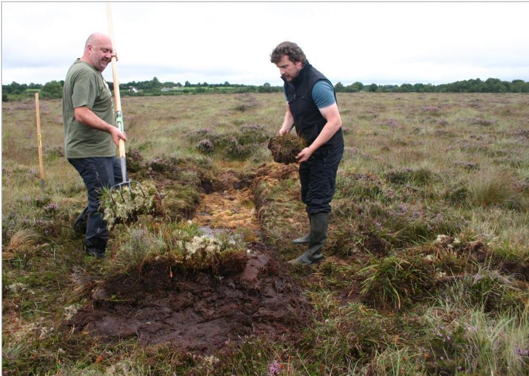
Figure 5.1 Example of a peat dam being constructed by hand © NPWS
